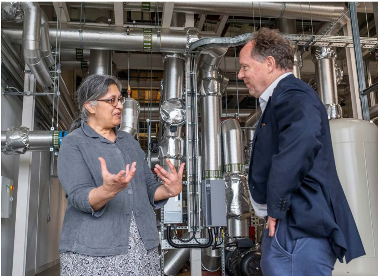
Commissioners tour Queens Quay Energy Centre, Clydebank
