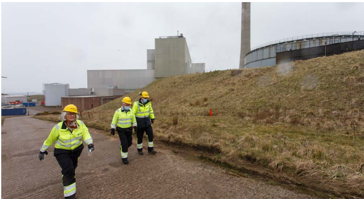
Commissioners visit the proposed site for a major carbon capture and storage facility adjacent to the existing Peterhead Power Station
