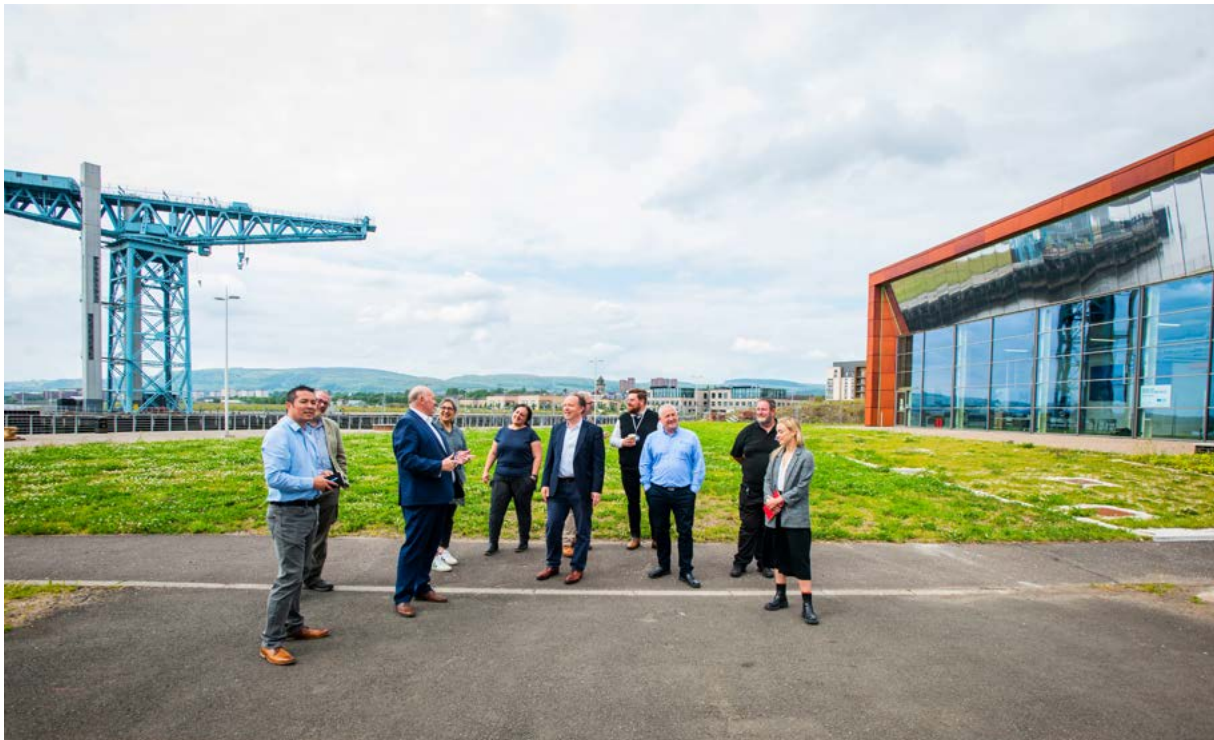
Commissioners stand between the Titan shipyard crane and Queens Quay Energy Centre, Clydebank
